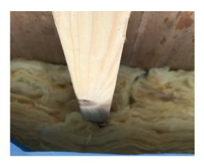
• With 8" joists the tabs will be stapled on the inside of the joist to maintain the insulation contact with the floor above.
